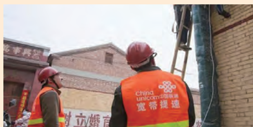
Rural network construction
