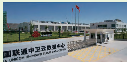
China Unicom Zhongwei Cloud Data Center
