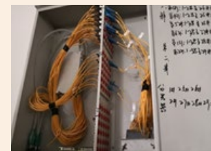
Rectification of network boxes and cable hubs.
