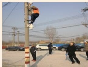
Removal of aerial "spider webs".
